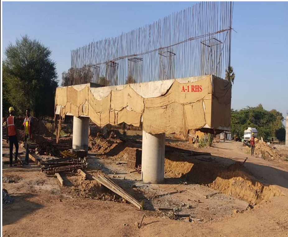
Abutment Cap –A-1 RHS A-1 side MJB @ 352+281
