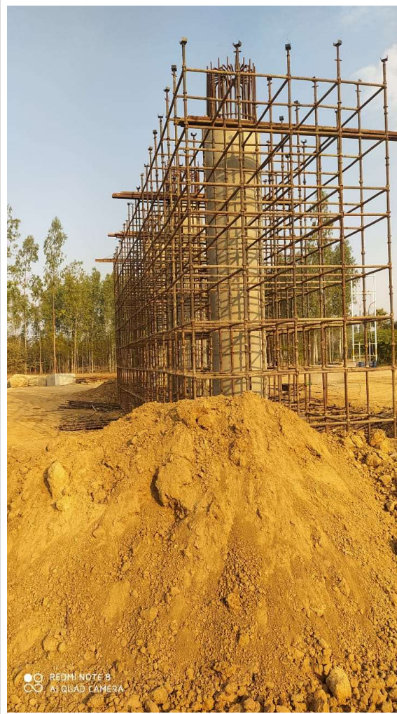
Staging & Shuttering Work for Pier Cap & Pier Shaft
