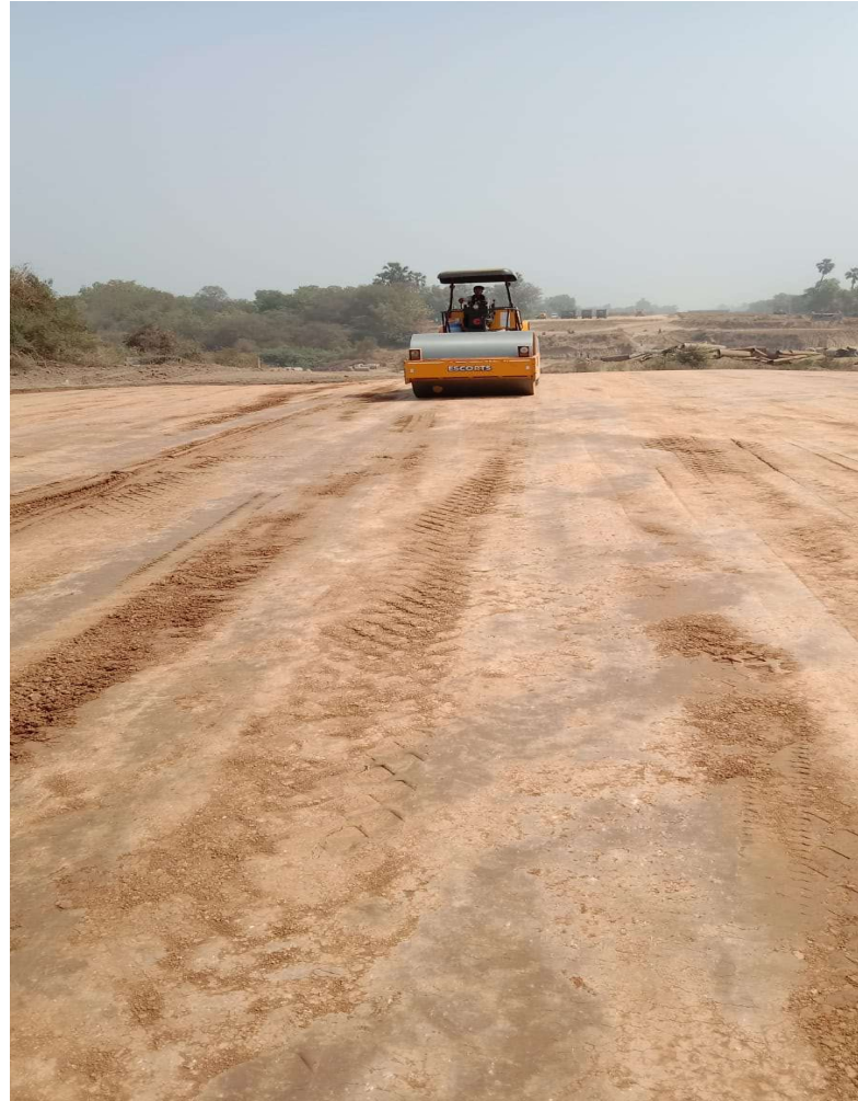
Embankment Rolling at site
