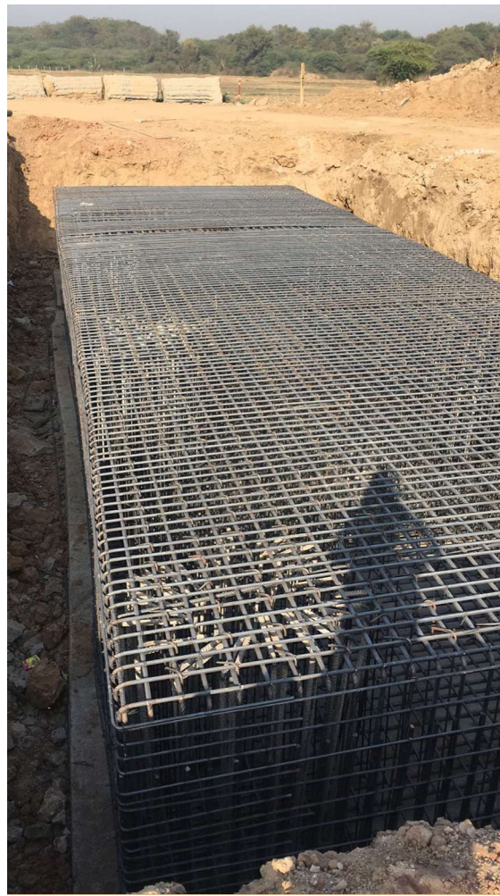
Pile Cap reinforcement binding work of Major Bridge
