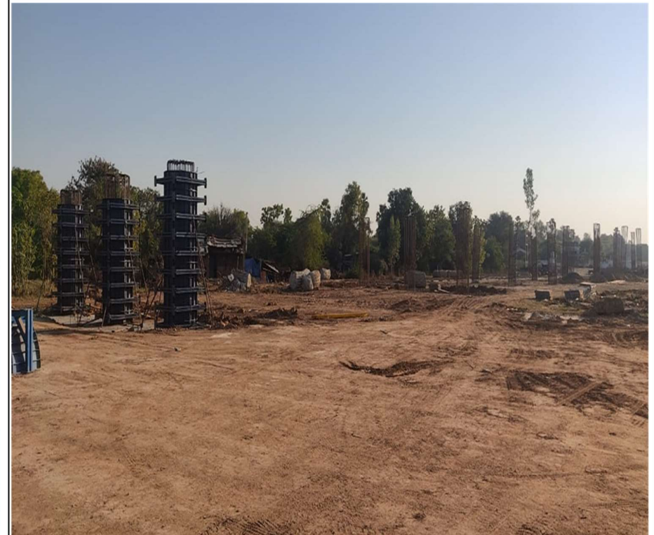
Pier Shaft A1 side LHS MJB @ 352+281
