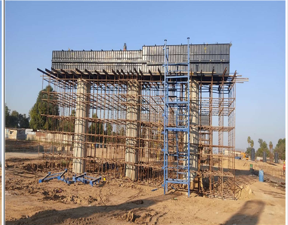
Pier Cap –P-5 RHS A-1 side MJB @ 352+281
