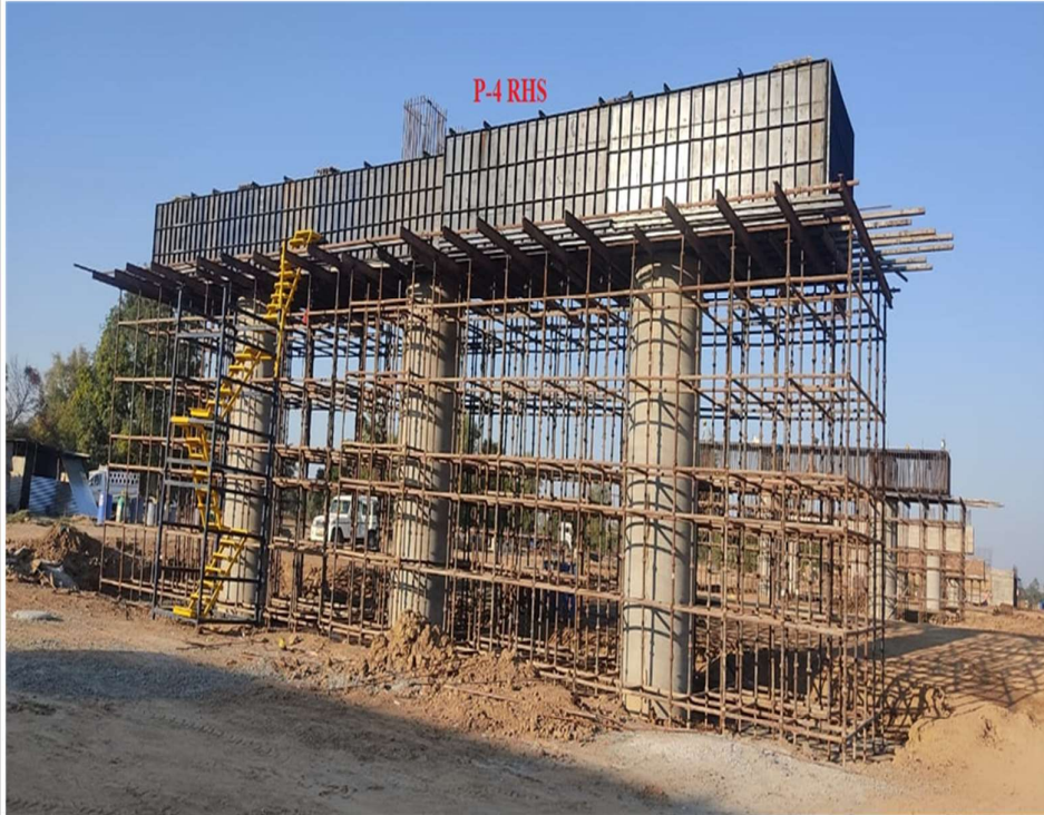
Pier Cap –P-4 RHS A-1 side MJB @ 352+281
