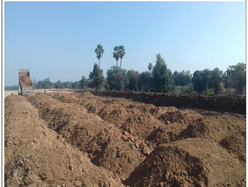
soil dumping In progress at ch.359+230 to 359+450 LHS
