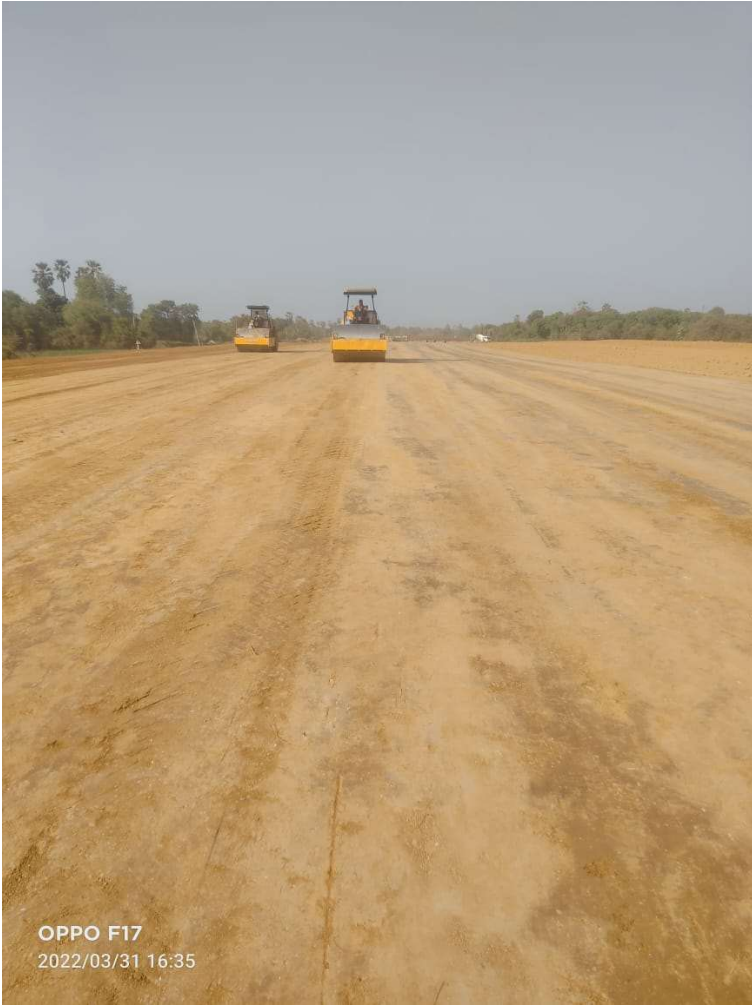
Sub grade Top Rolling work at site
