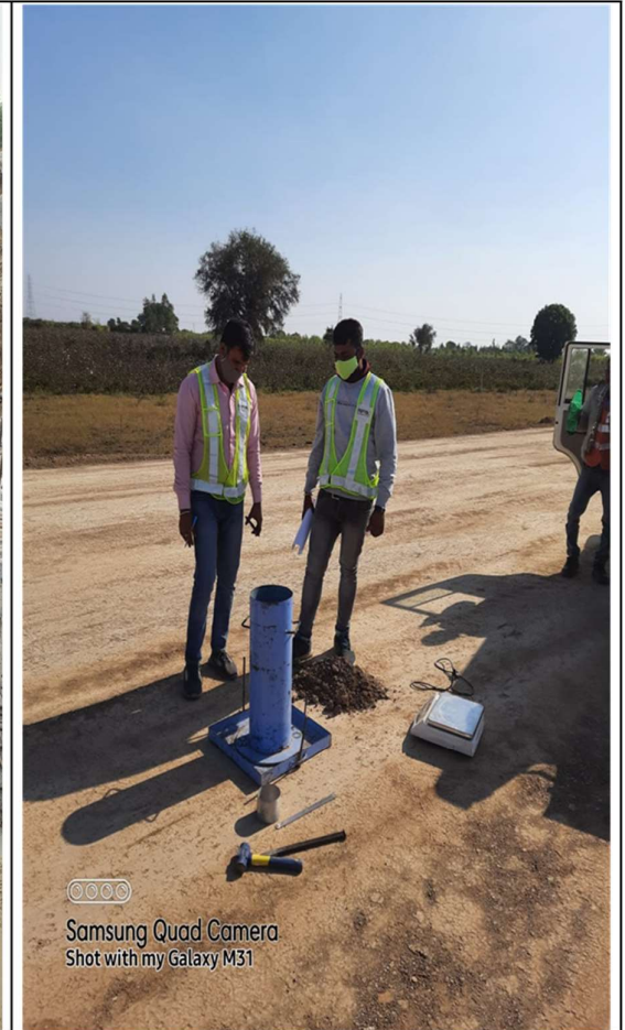
SG top fdd at ch.-360+ 600 to 360+ 720 LHS
