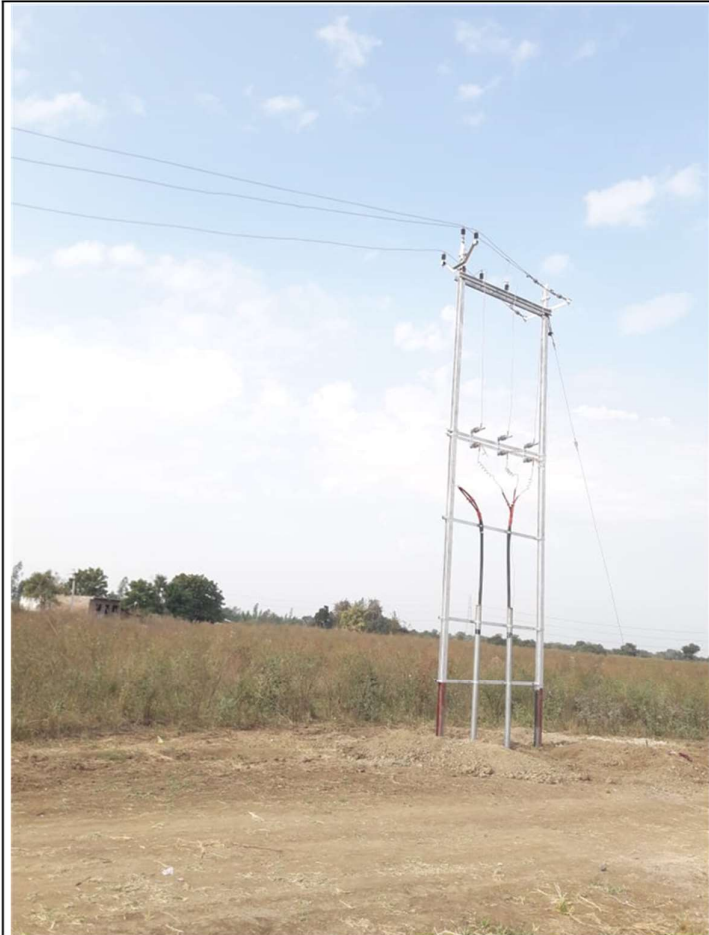
Utility Shifting- Electric line charging at ch.362+650
