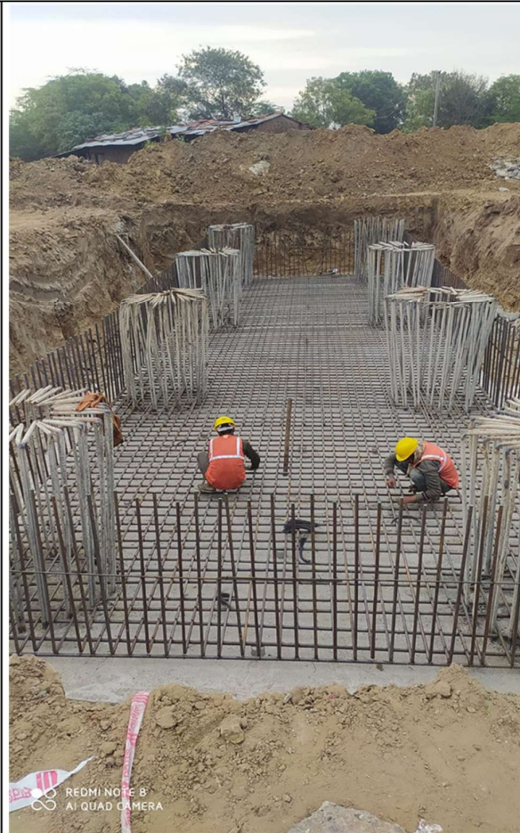
Pile Cap reinforcement binding at MJB 352+281
