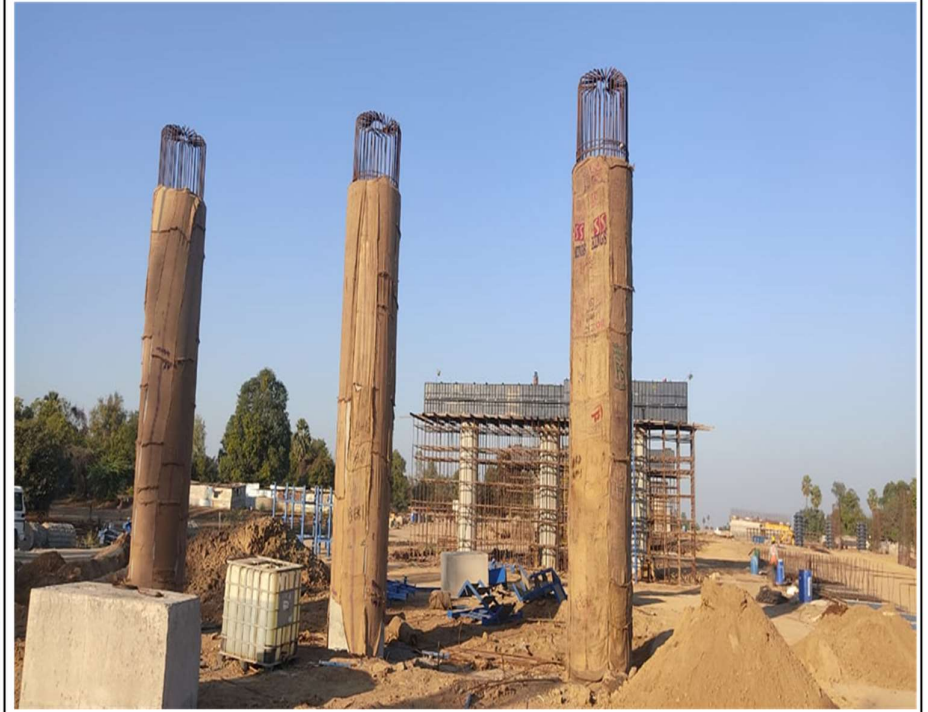
Pier Shaft P-6 & P-7 Curing A1 side at ch.-352+281 MJB
