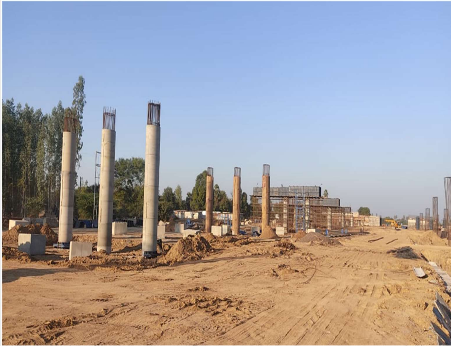
Pier Shaft P-6 & P-7 Curing A1 side at ch.-352+281 MJB
